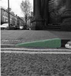
P1 Sloped Curb stone Time - 15:05 Location - Bedford Street
